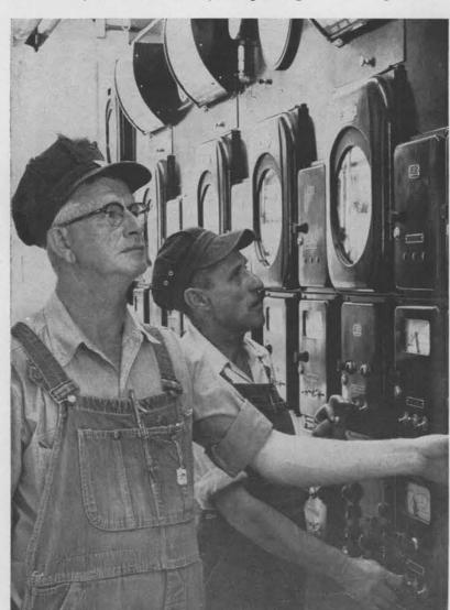
FUEL CHANGEOVER from gas to diesel is performed regularly for training purposes. In case of a gas failure, the steam plant could switch immediately to diesel. William Dickens, left, and Elbert Quail, boiler operators, man the damper controls during changeover.
